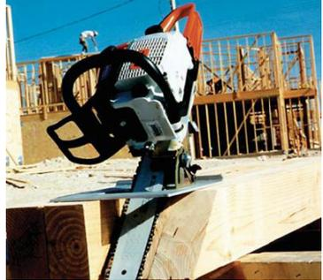
**5. Start the motor and place** the leading edge of the base plate on the top of the racked material just short of engaging the work with the saw chain. With the saw aligned to a snapped cut-line, or the base plate against a 2x4 guide fence, open the throttle and push the unit across the material until all the boards have been cut.
